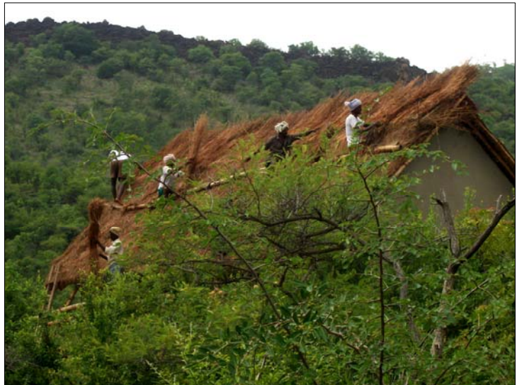
Use of local material for home construction Main policy of Timbaktu: live according to Nature, follow Nature, love Nature
