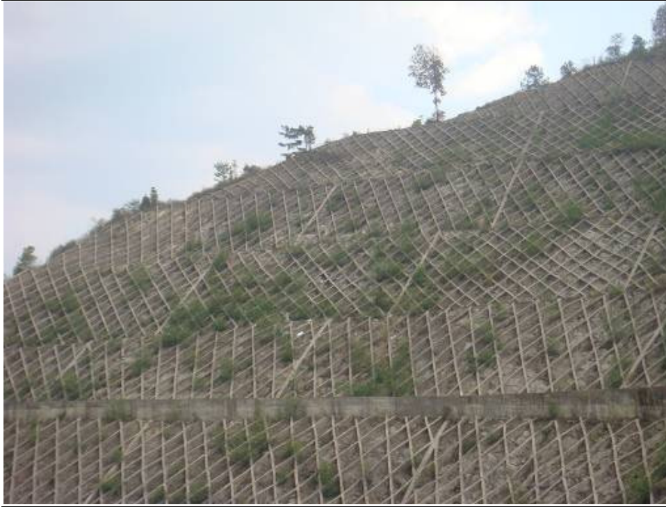
Photo 5 The reinforce concrete was poured on the mountain, in order to prevent water loos and soil erosion
