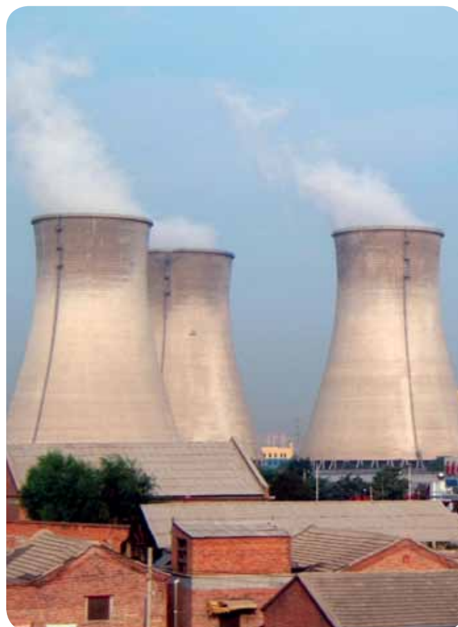
China Power Plant. Courtesy of Bret Arnett
