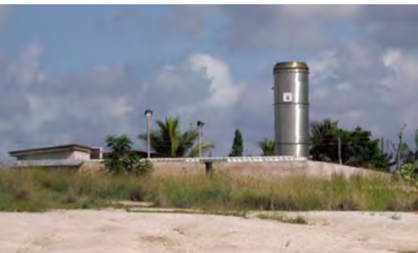
Mtoni landfill gas plant, courtesy of CSG
