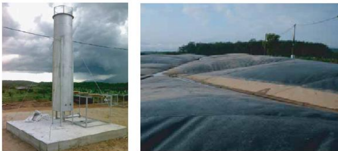
Figure 6. Foong Lee Mill - Flare (left) and methane collection (right)
