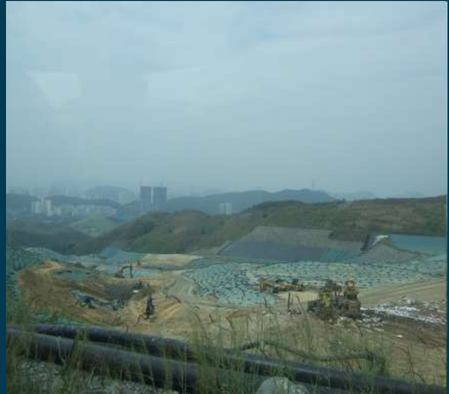
Sanitary Landfill with Landfill Gas Collection System under Construction (dwells and plumbing to collect the gas)
